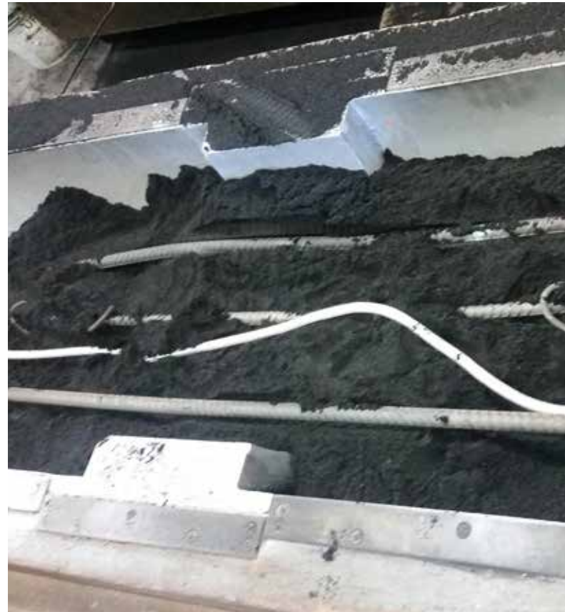
Vents placed into the core to create a path for the gases to exit without going into the casting.
